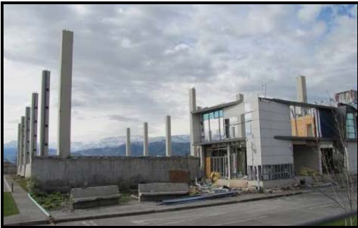
Damaged modern industrial facility (Lampa)
