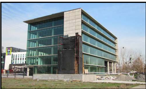
Office building repairs (Ciudad Empresarial)
