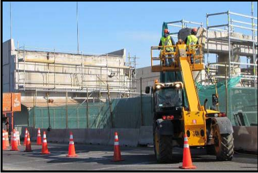
Bridge repairs (Vespucio Norte Highway)
