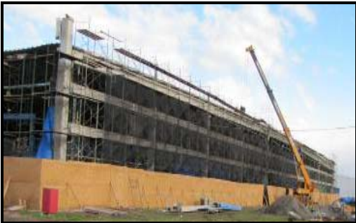
Repairs at a production plant (Lampa)
