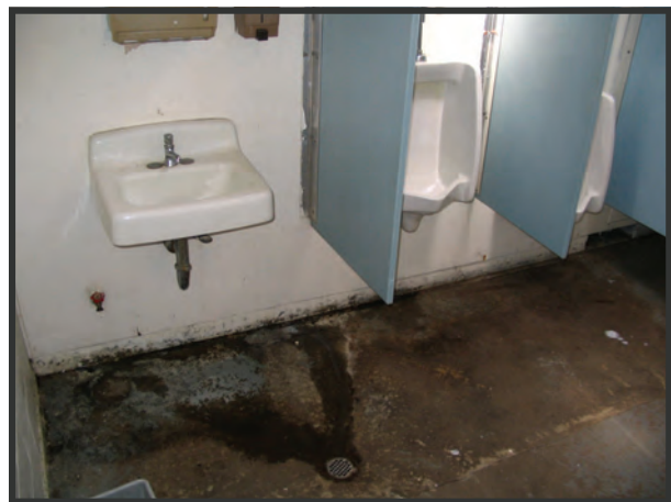
It is cheaper to let the Willamette Park bathrooms leak than to fix the plumbing.
