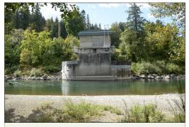
West Linn's water intake is on the Clackamas River. This state-of-the-art raw water intake withdraws water from the river and pumps it almost 2,000 ft. in distance and 300 ft. in elevation to the water treatment facility in Oregon City. The cities of West Linn and Oregon City have joint ownership of the South Fork Water Board.
