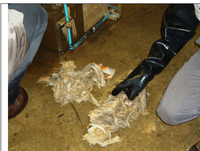
Photographic evidence of wipes in pipes.
