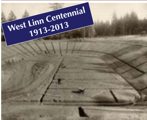
Bolton Reservoir construction in 1913. View this historic photograph and many others at WL100.org .
