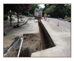
Following completion of water main improvements, the City's summer Road Program will repave the sections of roads impacted by the water main projects. By first replacing underground utilities and then repaving the full width of the road, motorists will have a smoother ride and there will be fewer trench patches, which helps to reduce the likelihood of new potholes forming.
