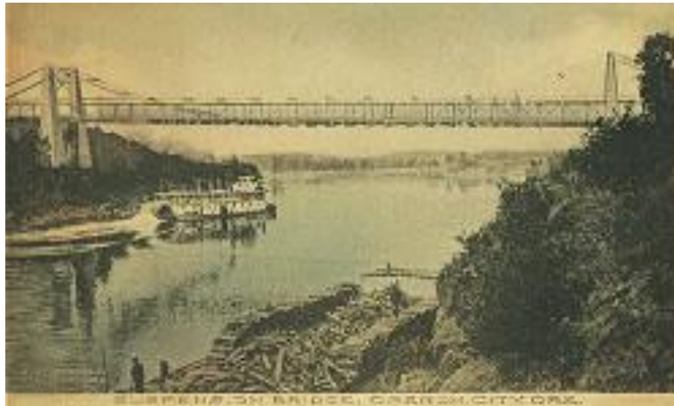
Oregon City Suspension bridge with ferry and Falls in background.
