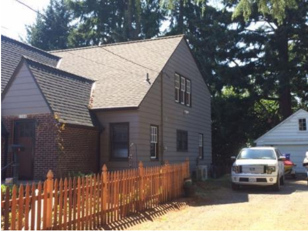
Side (north) Elevation – August 2014
