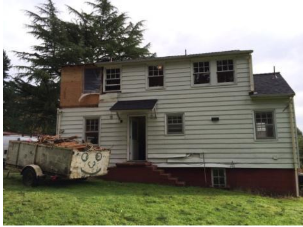
Rear elevation – October 2013
