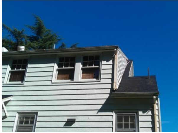
Rear elevation – September 2013
