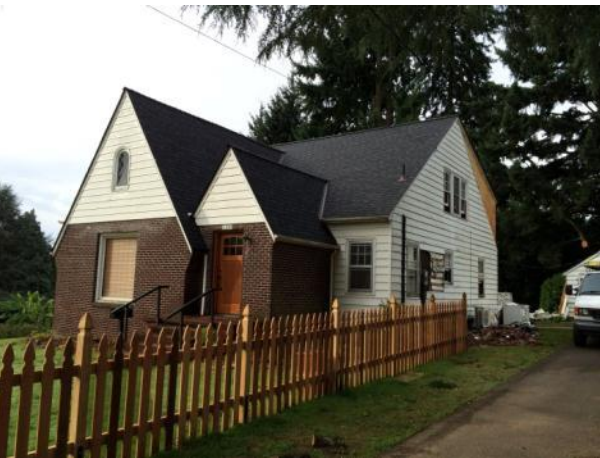
October 2013 – Front and side (north) elevation
