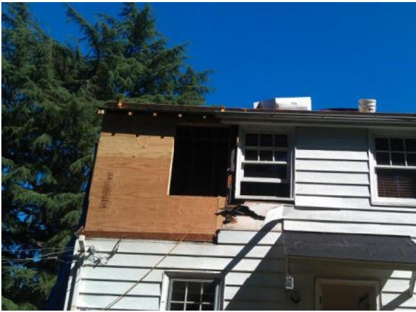
Rear elevation – September 2013
