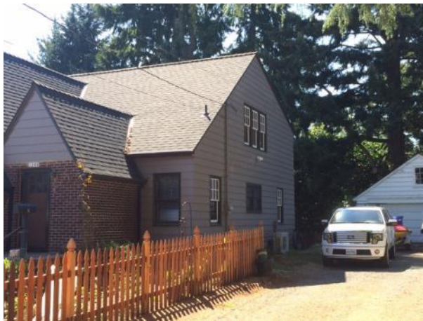
August 2014 – Side (north) elevation
