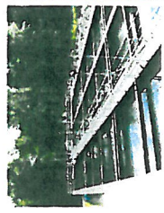
Lake Oswego Water Treatment Plant in West Linn
