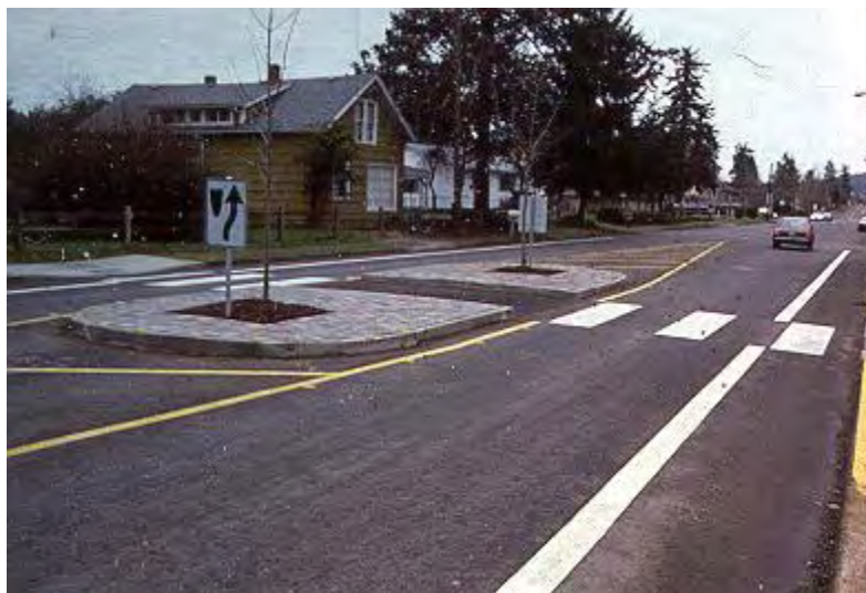
Figure 1: Example of Center Refuge Median on Two-Lane Street
