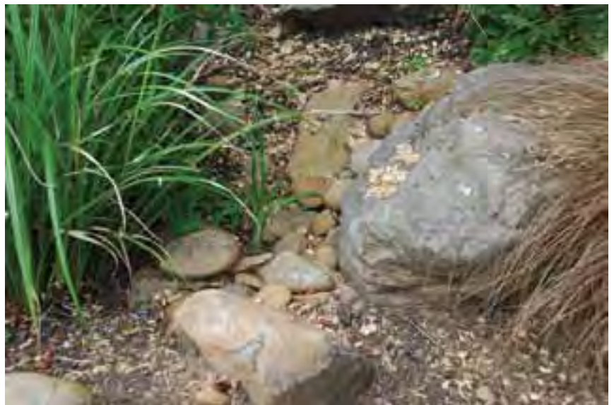
Figure 24: An outflow notch in a Portland, Oregon, rain garden, protected by rock to prevent soil erosion. (Photo: Robert Emanuel, OSU)
