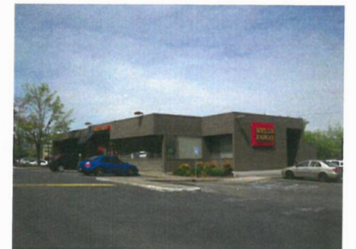
EXISTING IMAGE: Pad Building for Wells Fargo
