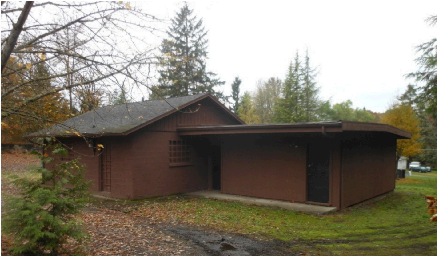
Figure 2-5: Building 2, The existing Water District Building
