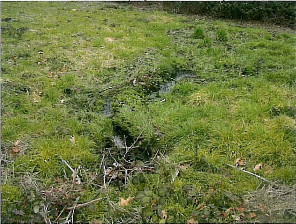
Photo W2 - Hidden Springs Stormwater Conveyance
