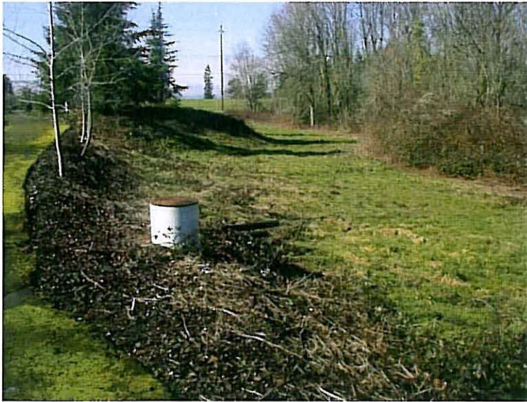
Photo 3 Hydrology alteration – Storm water drain pipe from Bay Meadows Drive subdivision
