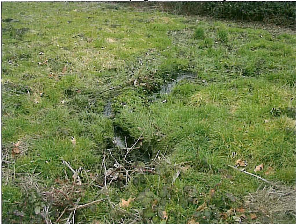
Photo W2 - Hidden Springs Stormwater Conveyance
