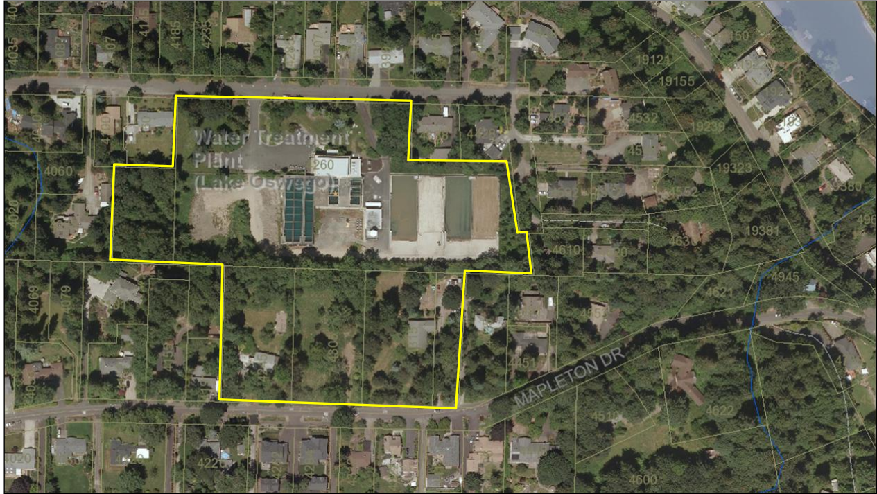
Figure 4: Aerial image of Applicant's site
