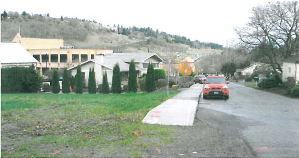
The photo above shows the view looking eastward on 8 th Avenue from the eastern end of the site. The Morton property buildings are in the foreground with the Willamette Marketplace's tan brick buildings in the background.
