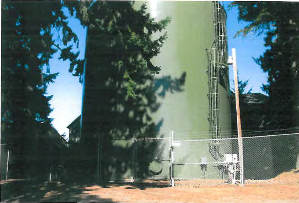
Existing reservoir on site, as seen from the south, from the area where pump station is proposed. The pump station is proposed to match the “forest green” color of the reservoir.
