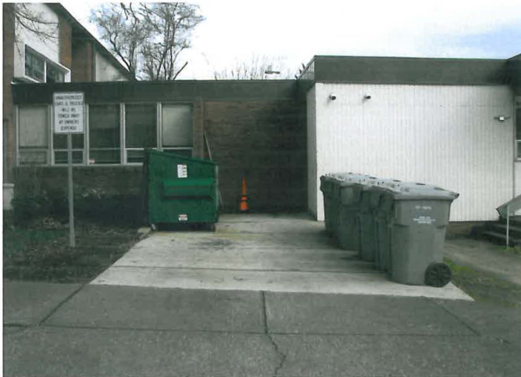
Trash/recycling area as it exists now. Cement area will contain trash compactor; gates will face street. To the left, in the background, the applicant proposes the masonry wall to screen the recycling containers and generator.
