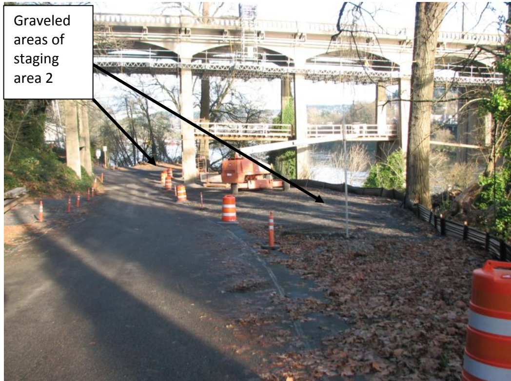
Lower staging area under the bridge along Territorial Drive
