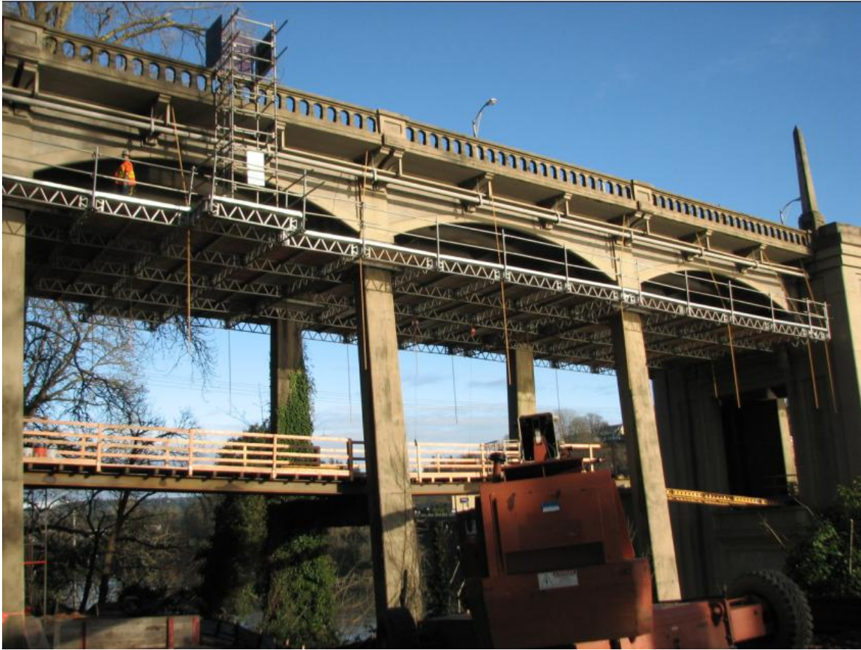
West Linn-Oregon City Bridge as seen from Territorial Drive/Staging Area 2
