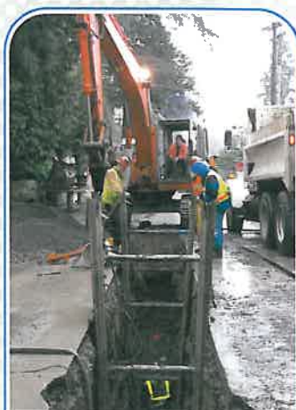
A crew may be able to install up to 100 feet of pipeline per day, depending on a variety of factors.
