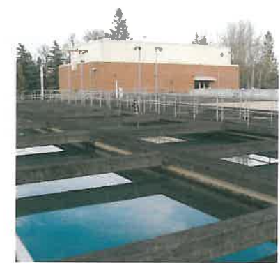
Lake Oswego's Water Treatment Plant in West Linn.
