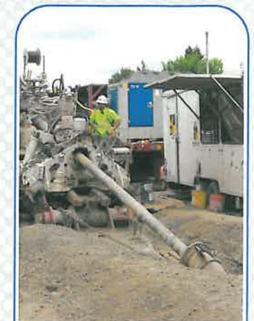
HDD uses a drilling rig on the surface to install a drill pipe in a shallow underground arc.
