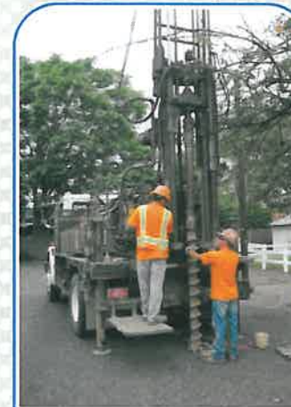
Crews conduct geological testing to determine soil conditions before pipe is installed.
