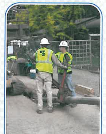
HDD crew at the exit point for the installed pipe.
