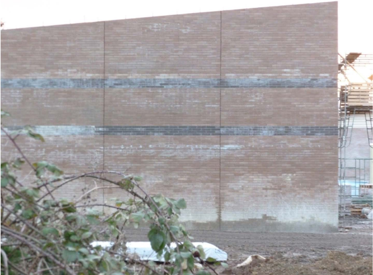
The efflorescence on the play structure detracts from the neighborhood. The notion of 'white elephant' comes to mind. Unmentioned is the reverberation and noise levels of the busses turning around less than 50 feet away from the Covered Play Structure. If I lived in one of those homes in the background, I would not be so polite as I have been in this missive. Even if this meets seismic requirements, I hope I am not under the structure when a Fukushima-like earthquake hits the Northwest! And our kids are supposed to play around this monstrosity? Welcome to the Hindenberg, kids!
