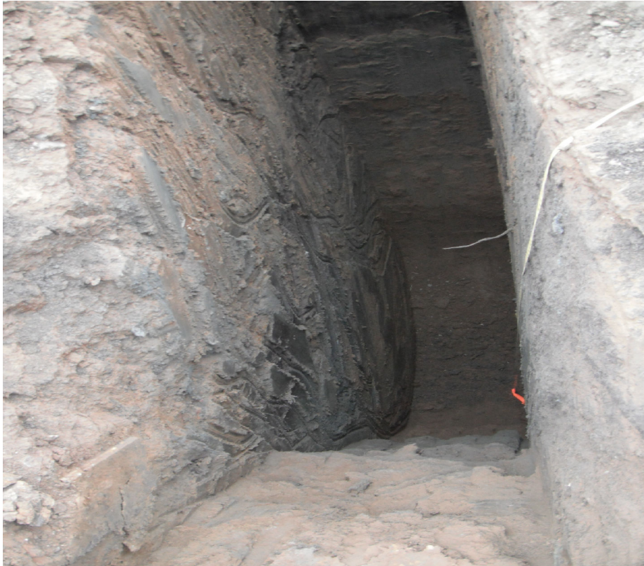
Photograph 1: Test pit TP-1 excavated depth 0 to 15.5'
