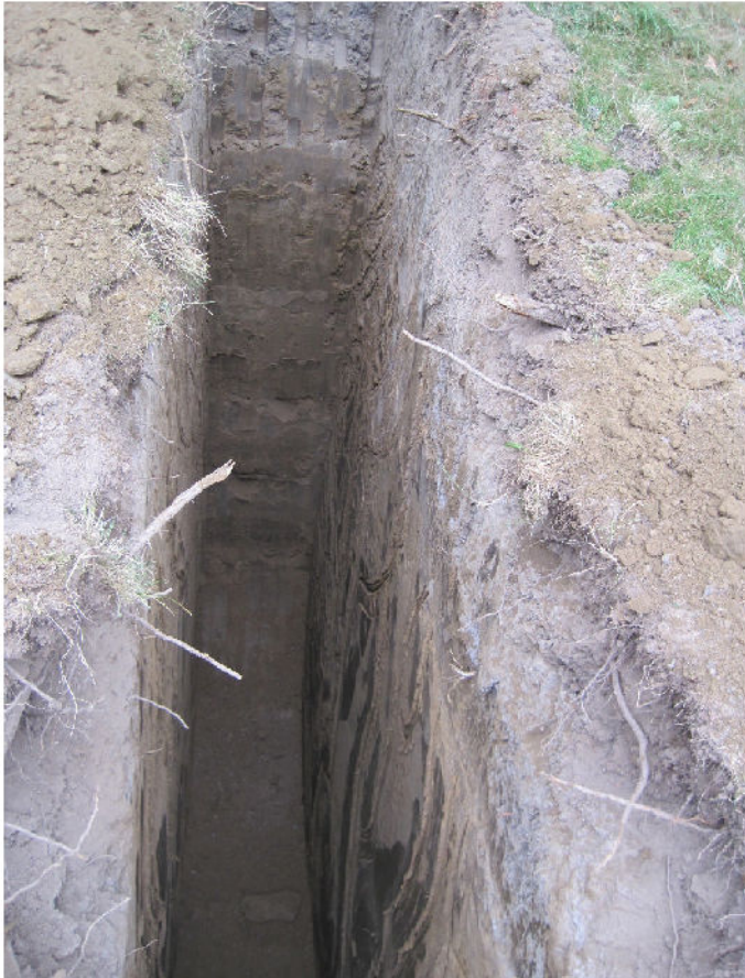
Photograph 7: Test pit TP-4 excavated depth 0 to 14.5'
