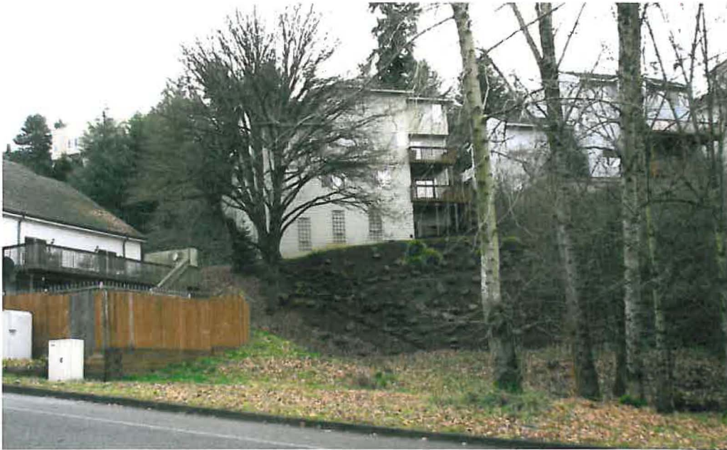
Houses on west end of Greene Street, with Tannler Drive in the foreground. These properties back up to the north end of the site, near where the northern trailhead is proposed.
