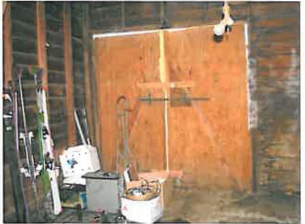
Interior View, garage door
