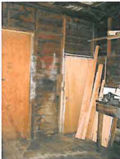
Interior view, garage and man door
