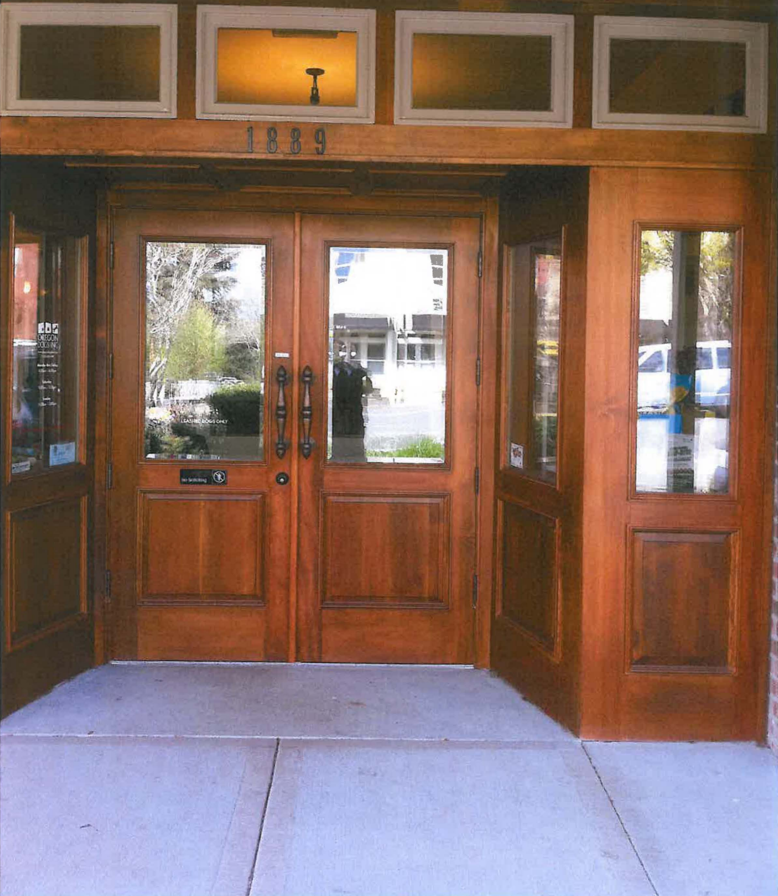
Photo #5 – 1823 proposed doors and stained window/door trim
