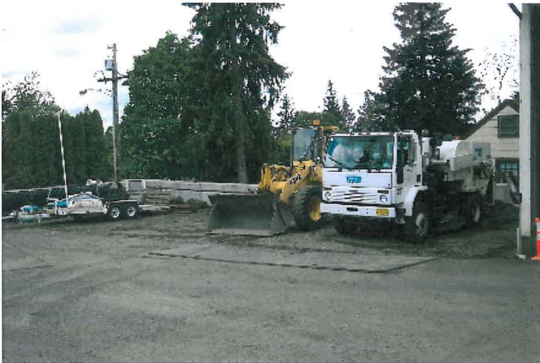
Covered Parking Building Site – Looking Southeast
