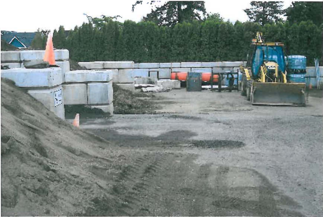
Materials Storage – Looking East
