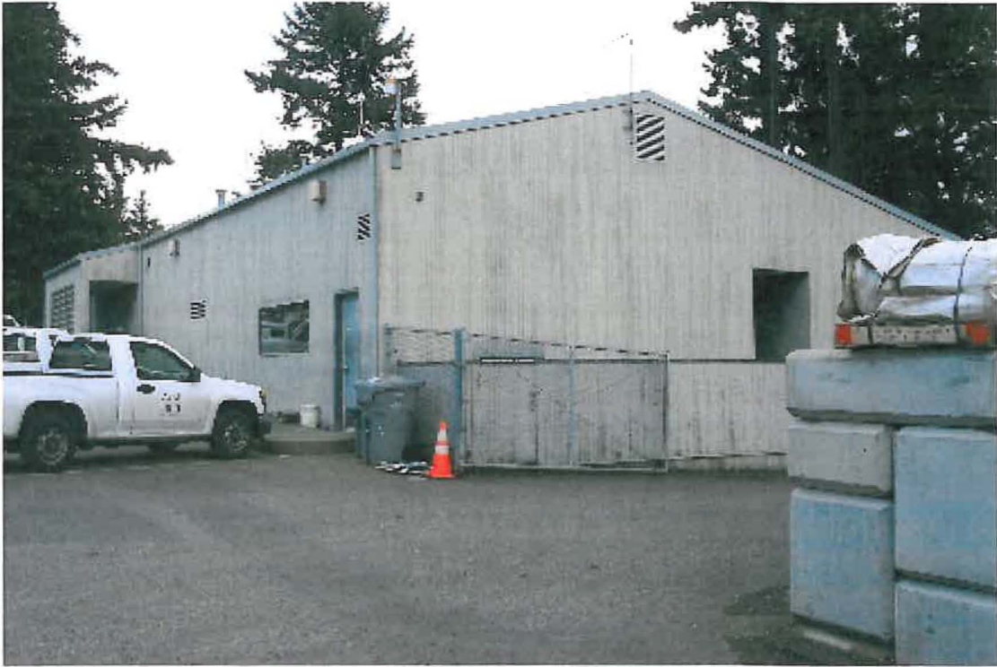
Administration Building – Looking Northeast
