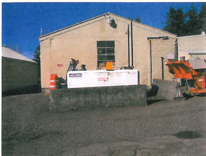
Fuel tank area existing conditions
