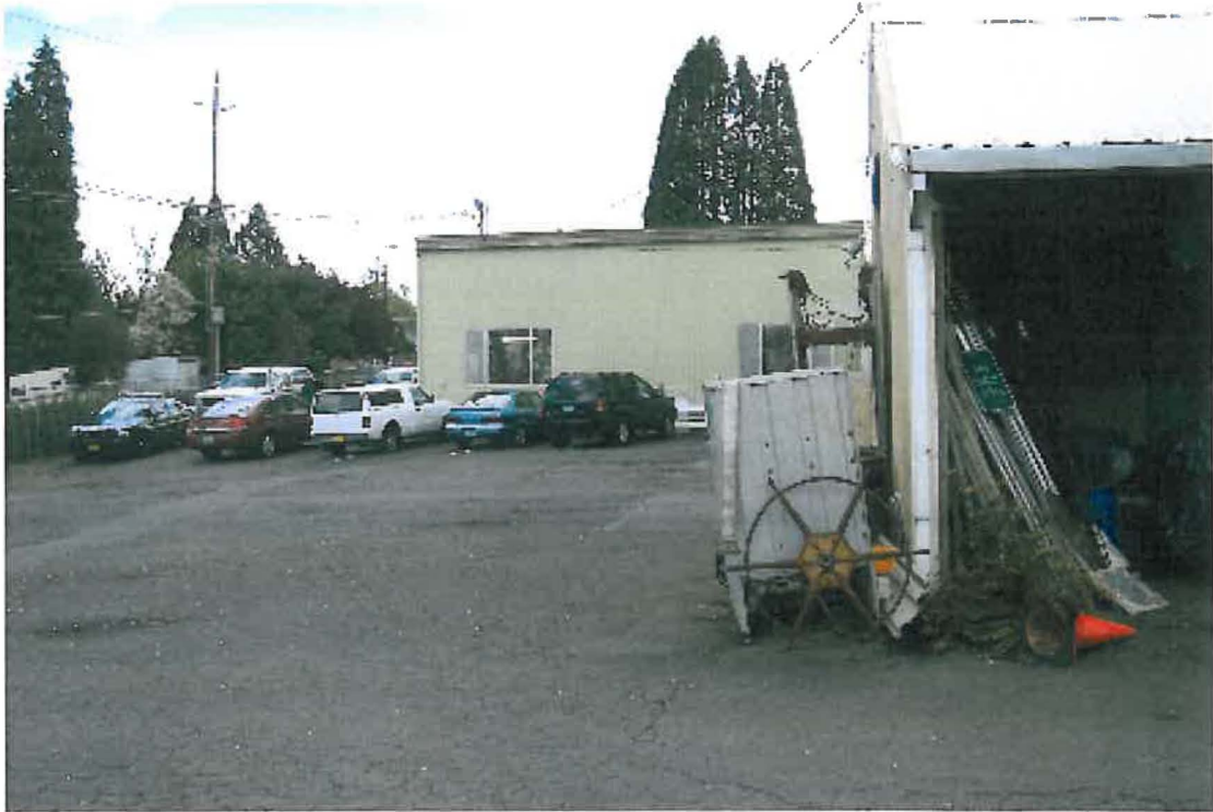
Vehicle Maintenance Shops – Looking North
