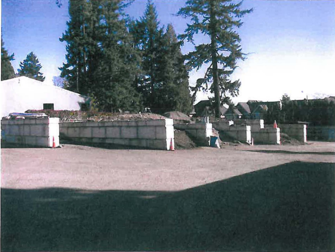
Inside of materials storage area, including walls that have not gone through design review yet
