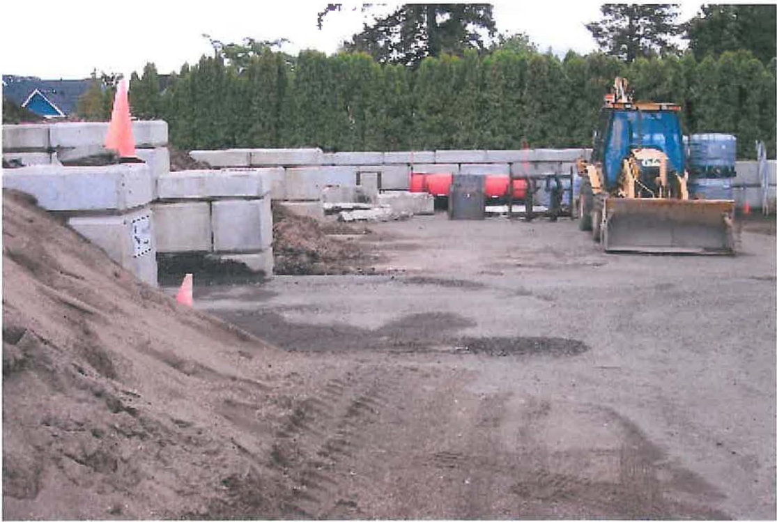
Materials Storage – Looking East
