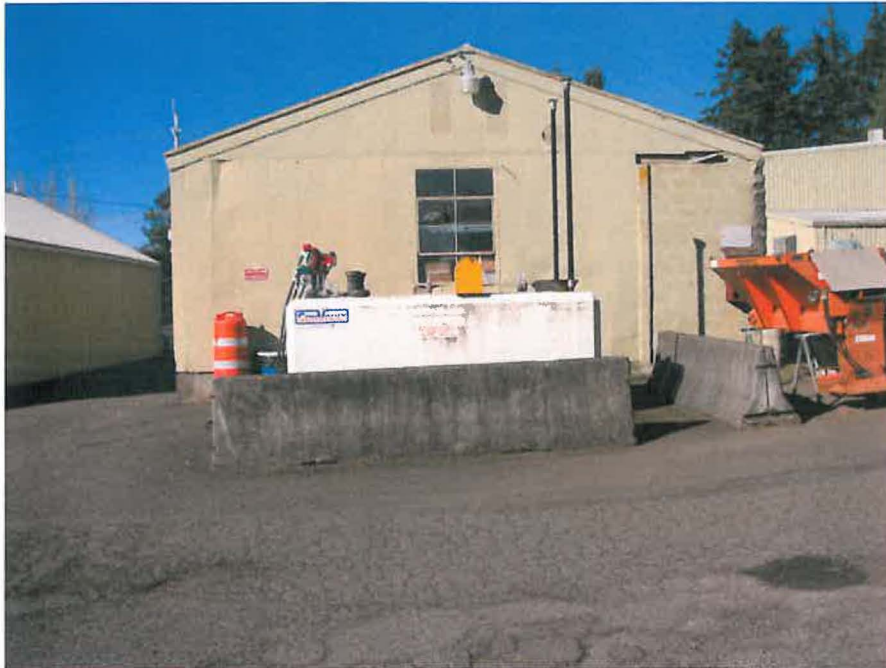
Fuel tank area existing conditions
