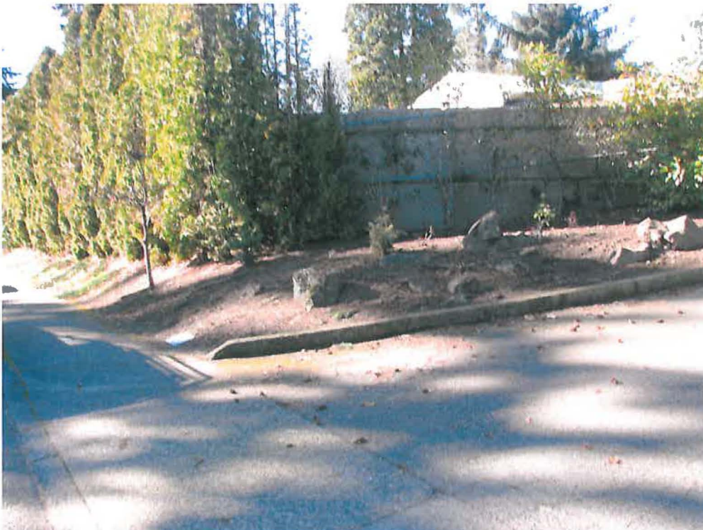
Area by Public Works driveway entrance where not-yet-reviewed walls are visible
