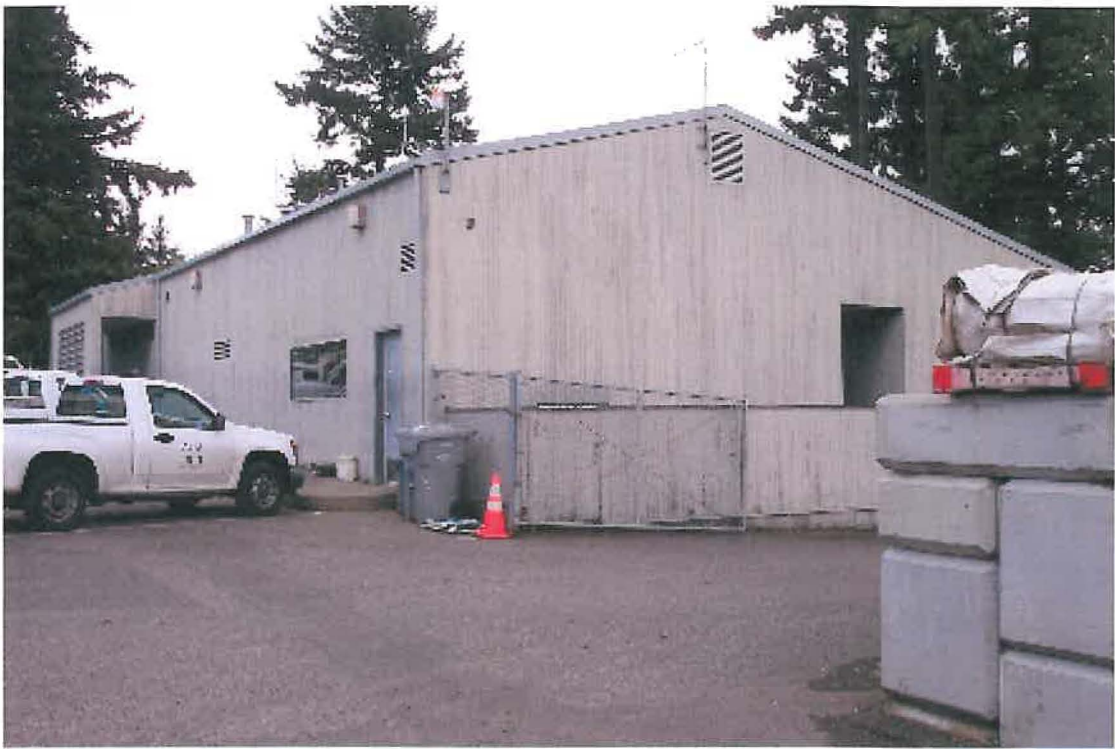
Administration Building – Looking Northeast
