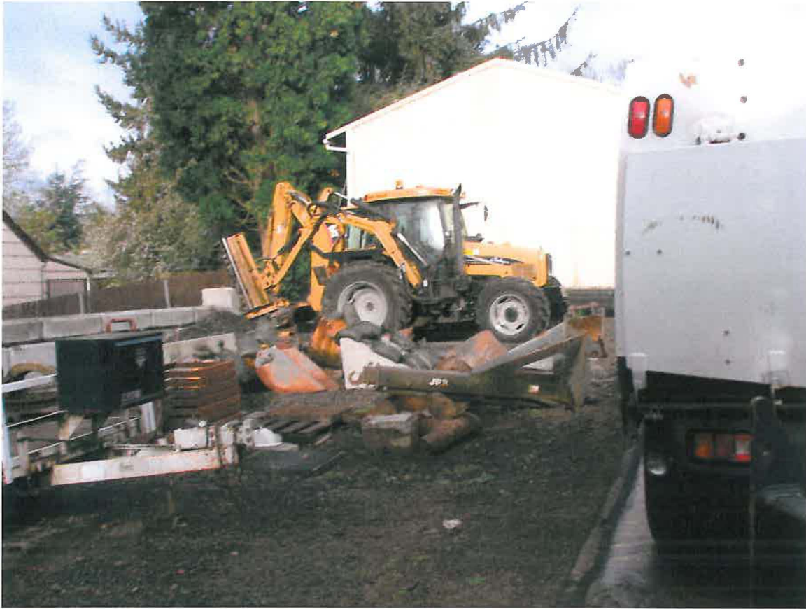
Location where new vehicle shed is proposed in materials storage area. Existing vehicle shed is in background to the west.
