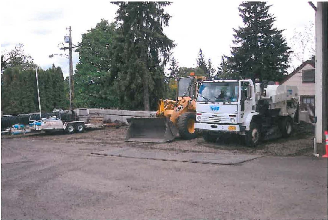
Covered Parking Building Site – Looking Southeast
