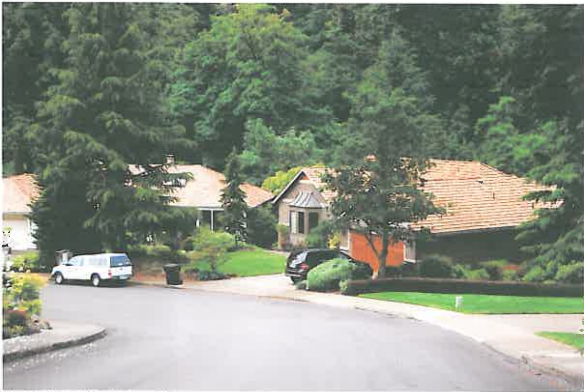
Photo 10 – Fire Haz - River front homes with cedar roofs in Swift Shore development.
