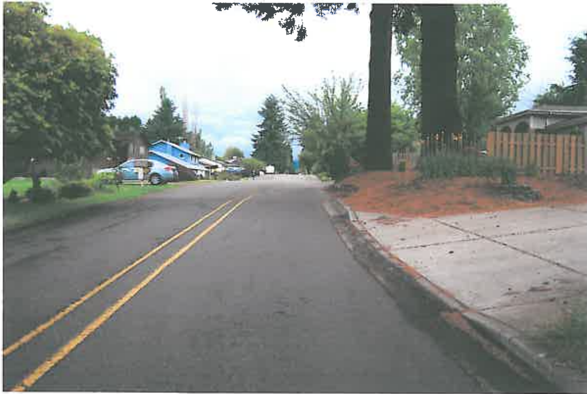
Photo 1 –Safety issue @ 1780 Ostman Rd –Hill crest, Tri-met route, 8' wide lane.
