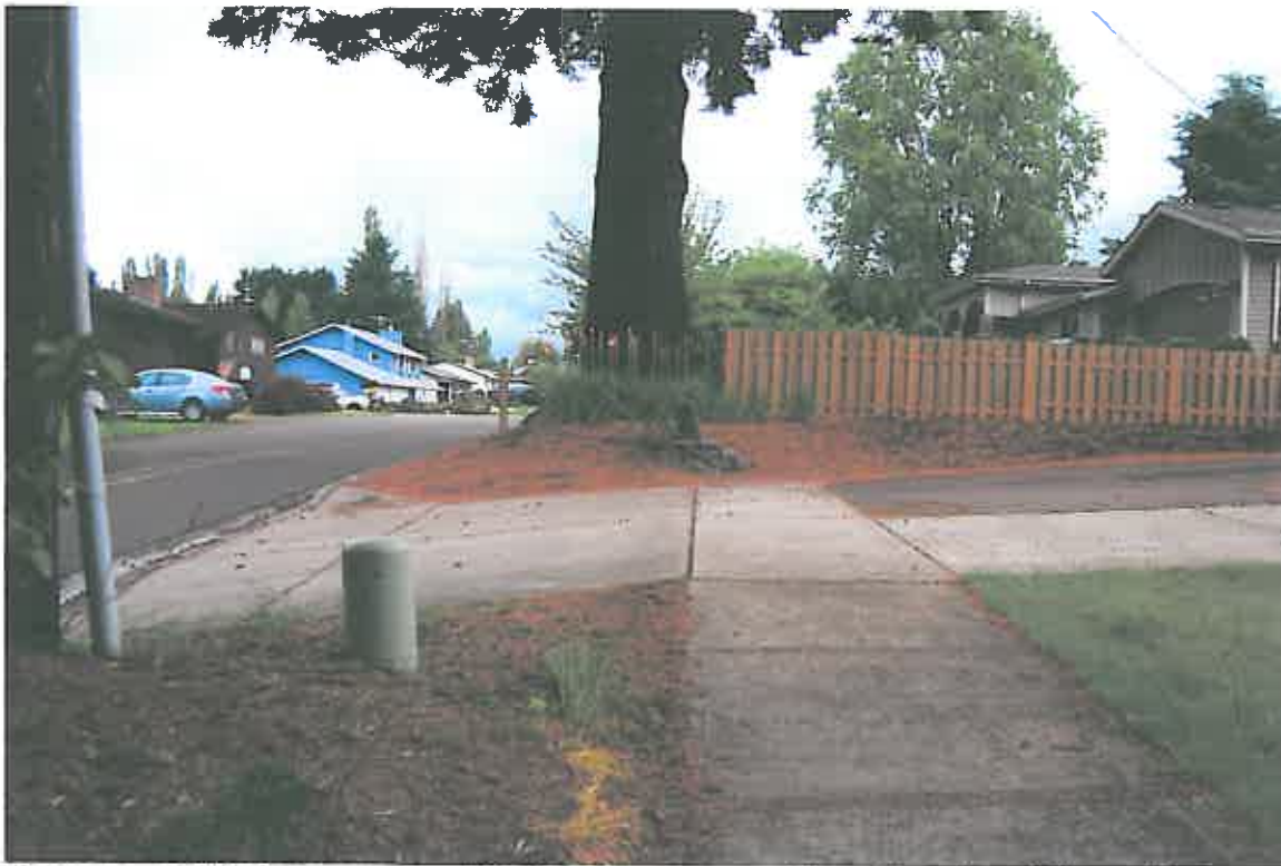
Photo 2 – 1780 Ostman Road Safety issue – no sidewalk and no bike path.
