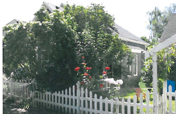
Side (west) Façade
