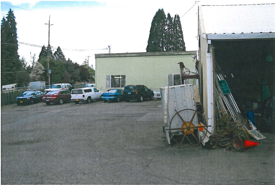
Vehicle Maintenance Shops – Looking North
