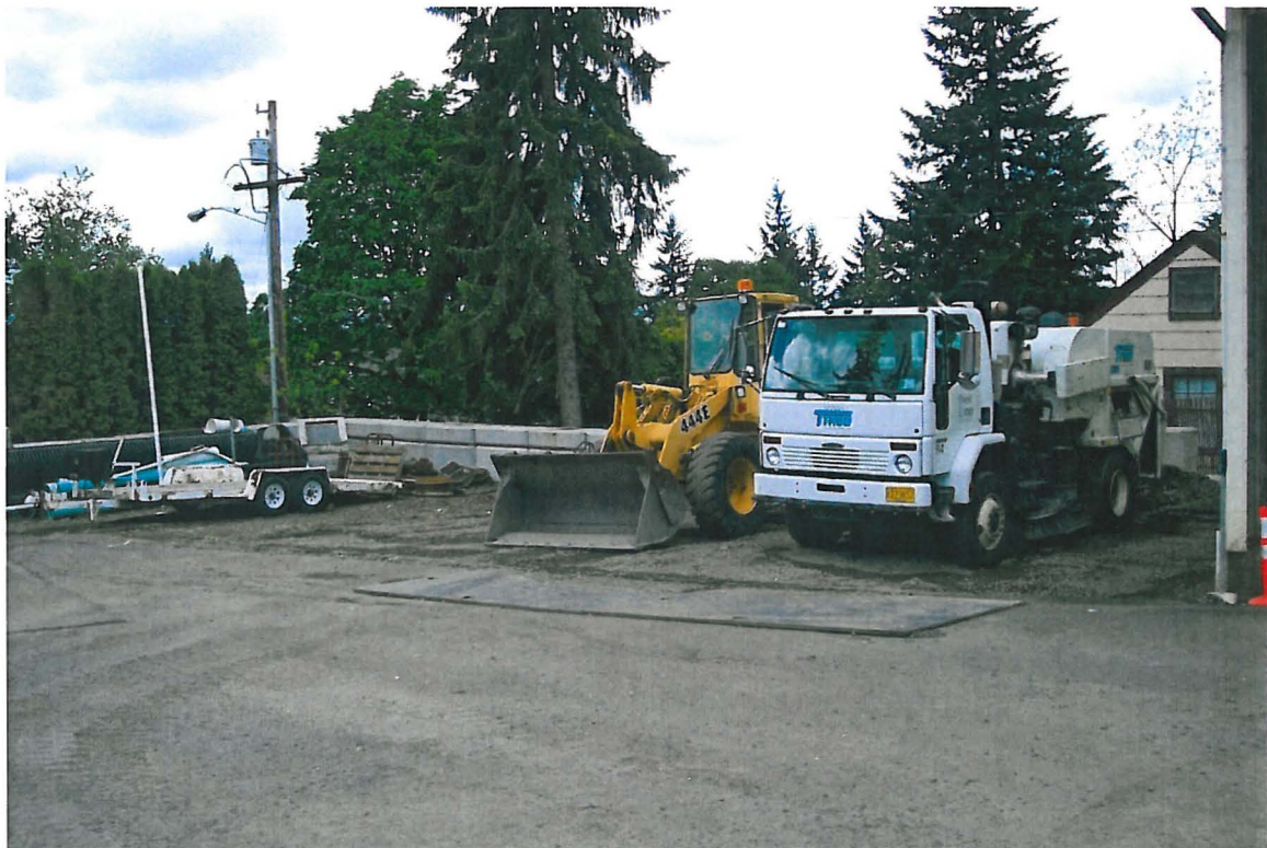
Covered Parking Building Site – Looking Southeast
