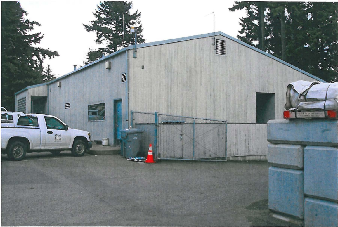
Administration Building – Looking Northeast
