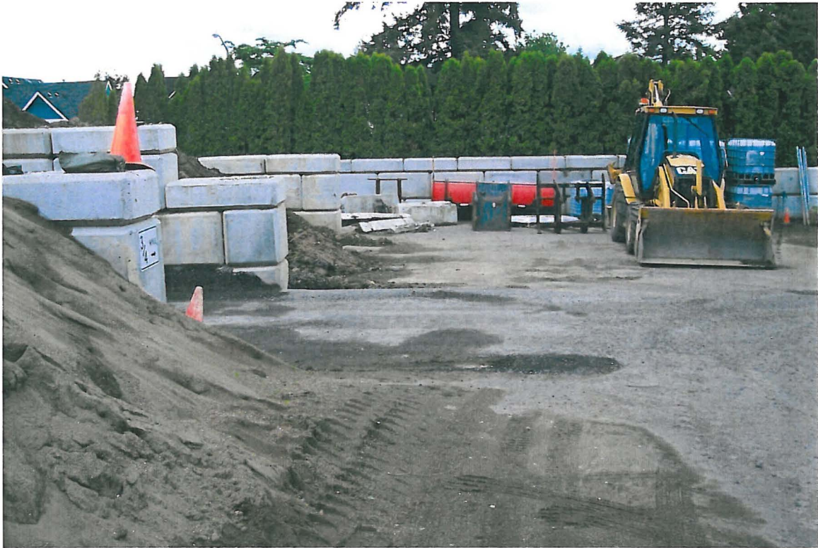
Materials Storage – Looking East
