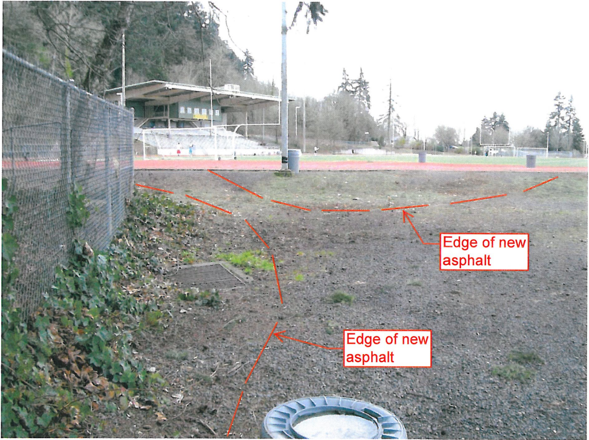
Existing gravel area to be overlaid with asphalt. (west portion)
