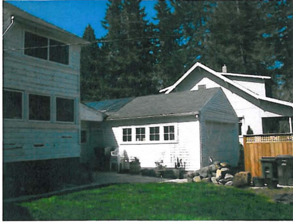
Side yard view of existing rear addition and garage
