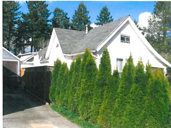
Side (northeast) elevation
