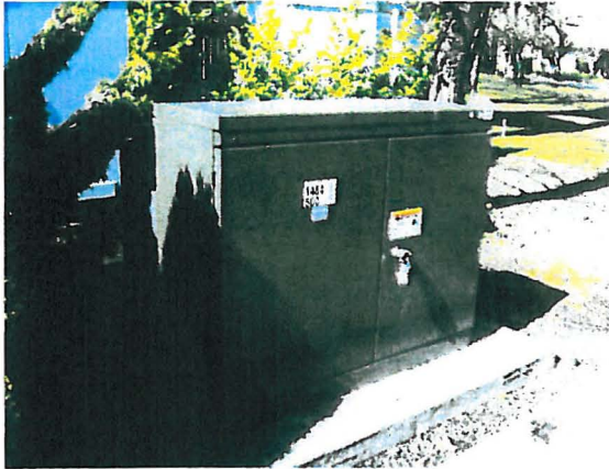
Photo #9 A pad mounted transformer southeast of the site area.
