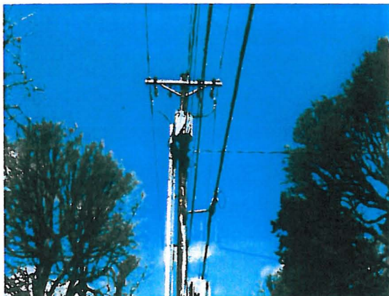
Photo #11 A pole mounted transformer directly east of the site area.
