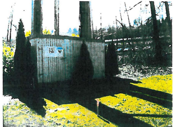
Photo #2 Looking south across site.
