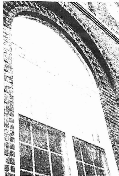
Newly painted double-hung wood windows.
