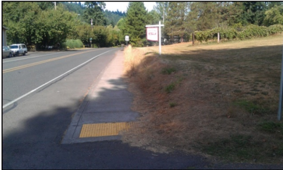
Willamette Falls Drive frontage
