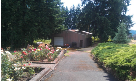
Existing pole barn and garden
