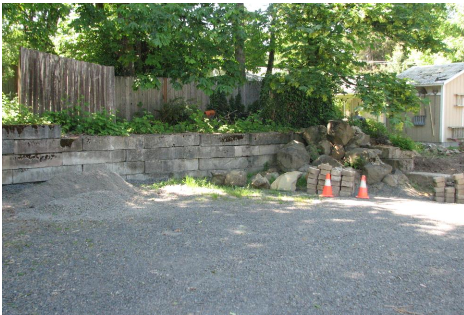
Western edge of parking lot
