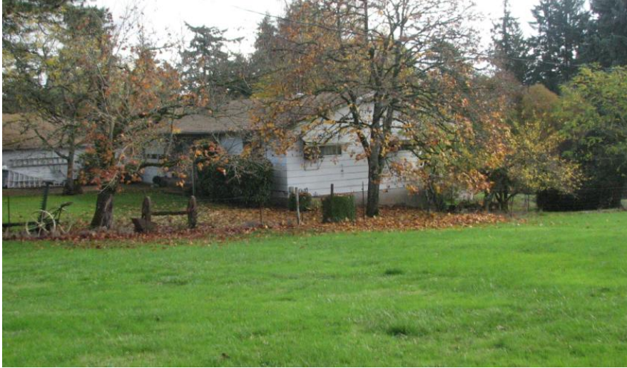
House at 20800 Hidden Springs Road
