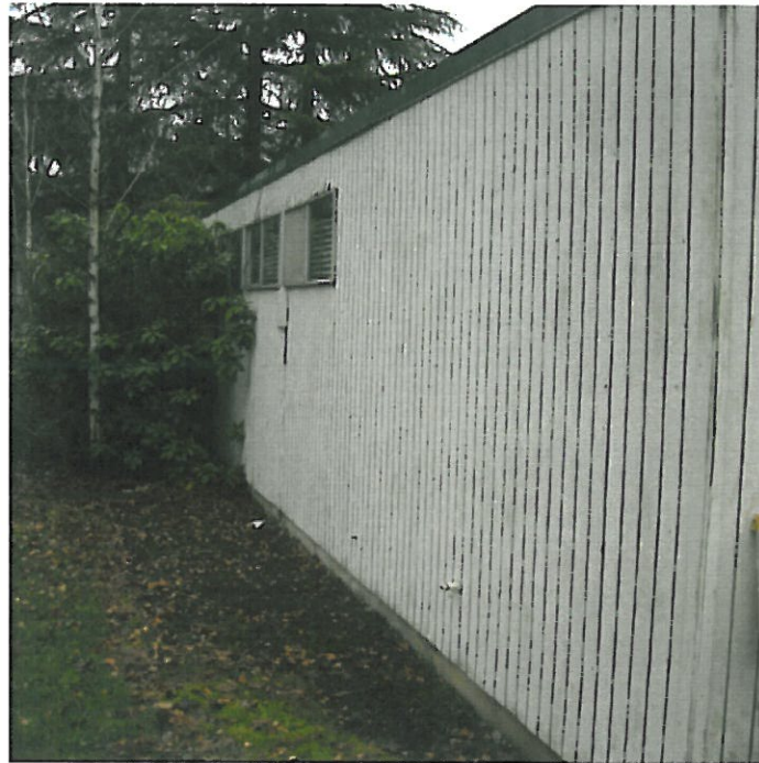
Figure 3: Exterior Wall, West
