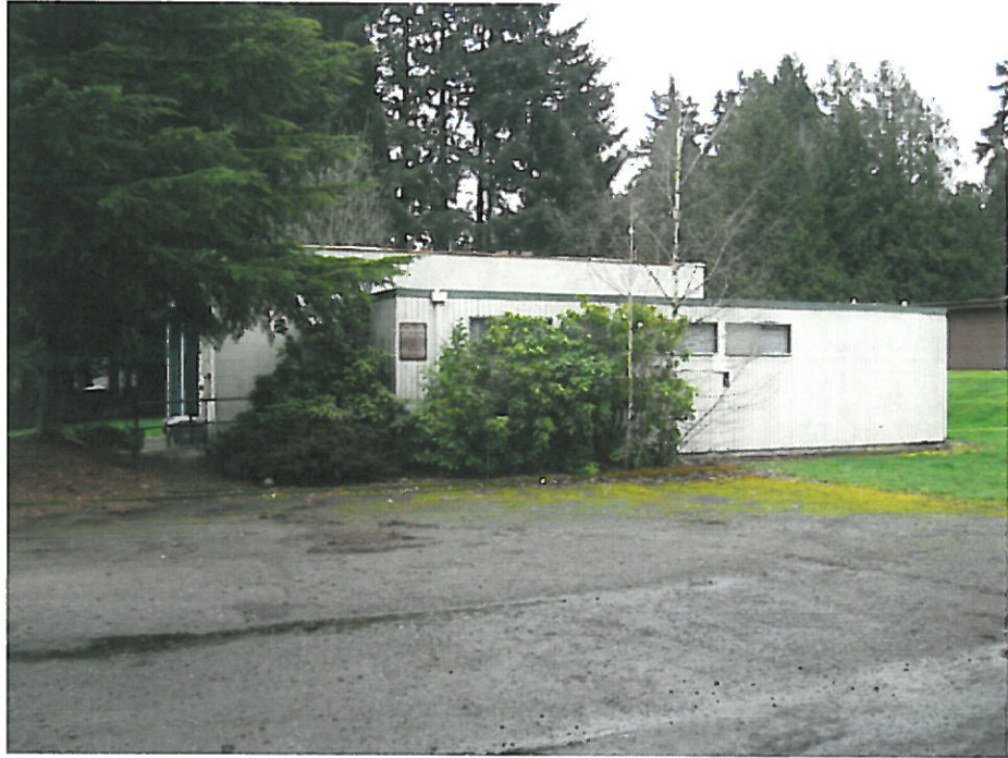
Figure 1: Parking Area, West Facade
