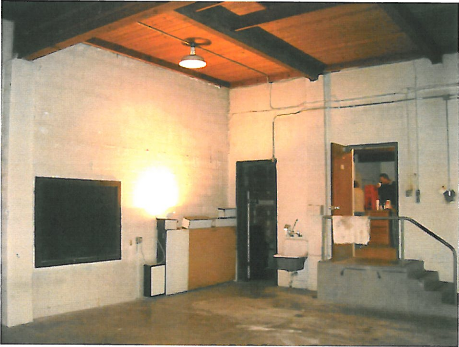
Figure 7: Garage Bay, Rear
