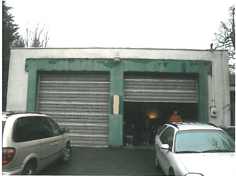
Figure 5: Garage Bay, North Facade
