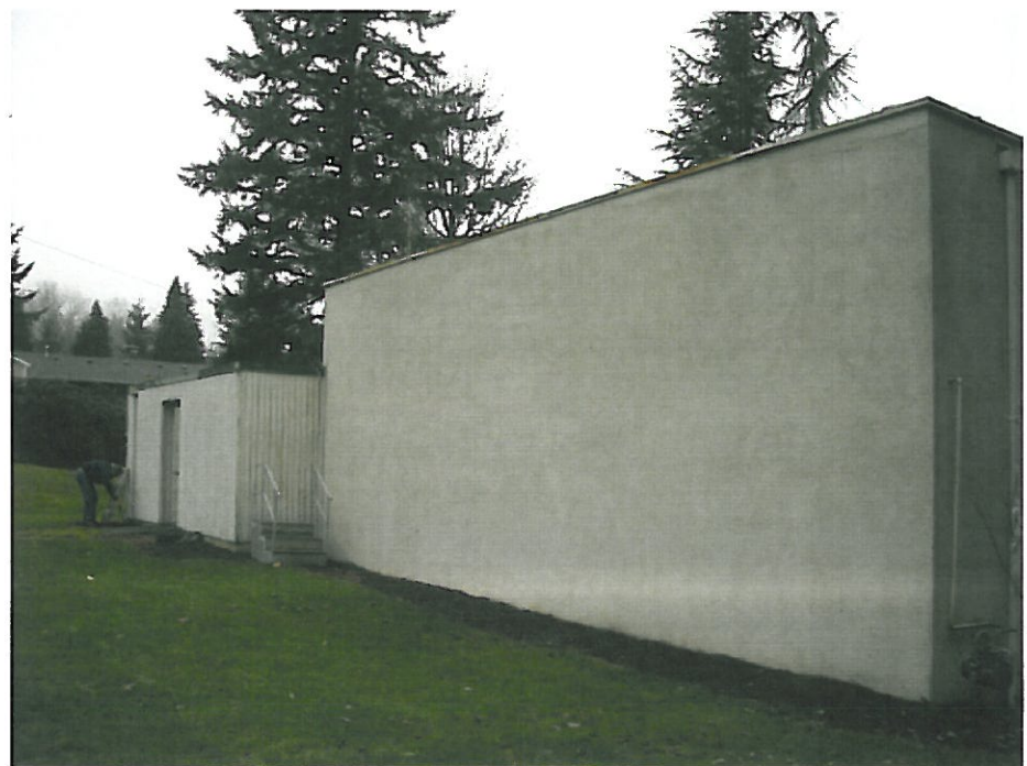
Figure 4: Exterior Wall, South
