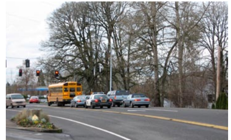
This curb/median prevents left turning movements to/from this shopping center driveway; shoppers instead must use the left turn lane and signal at the Hidden Springs intersection
