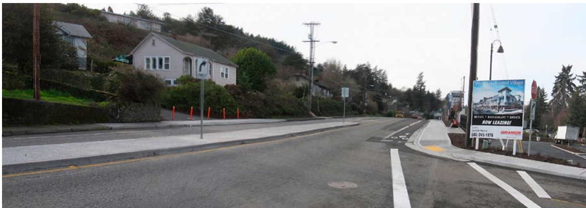
This substantial median prevents left turning movements to/from the Central Village Development; patrons are thus directed to the signalized intersection at Hood/McKillican
