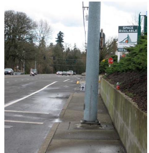
This image contains a particularly ironic example - a light pole (with pedestrian crossing button) that blocks access to a crosswalk curb ramp
