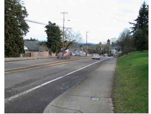
Steep slopes adjacent to and within the right-of-way sometimes limit the ability to expand existing facilities or provide new ones
