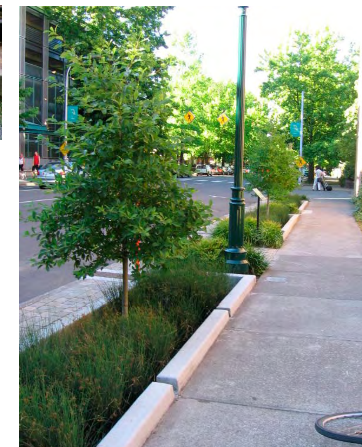
Stormwater planters are often linked together, so that when one planter fills up, water flows down into the next planter
