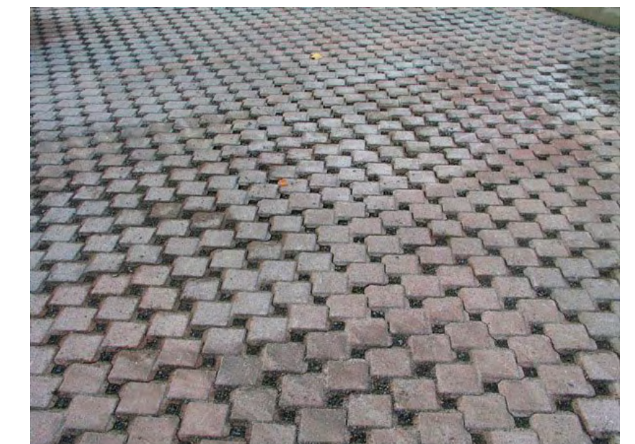
Porous paving within the on-street parking strip serves both to define the parking area as distinct from the rest of the right-of-way, and manage stormwater runoff
