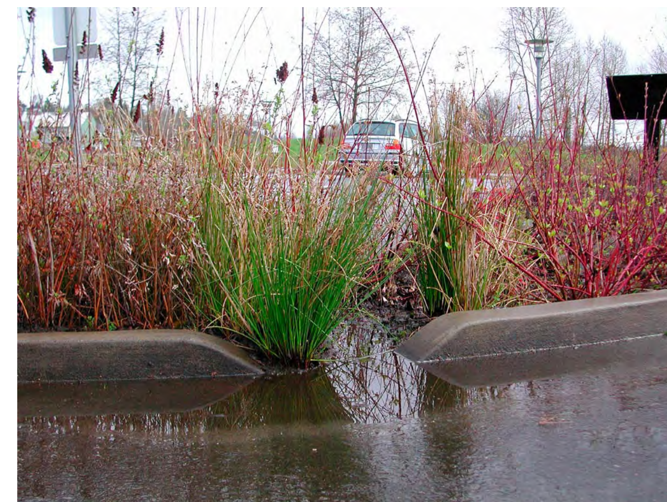
Slotted curbs direct water into the planter, where it is allowed to collect and eventually seep into the ground
