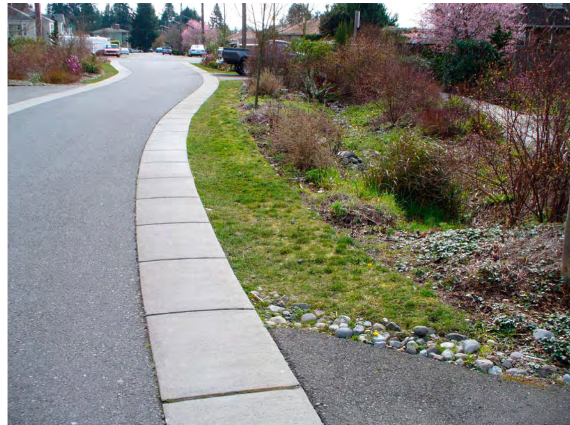
Paving treatments can be used to visually define the edge of the street in the absence of curbs
