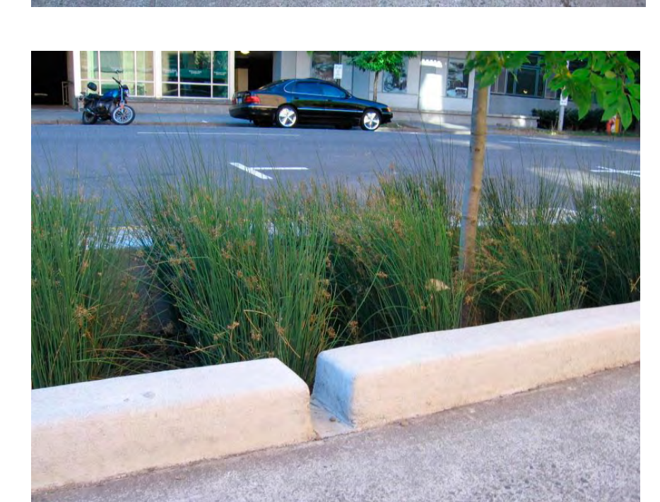
A slotted curb adjacent to the sidewalk allows the planter to collect runoff from sidewalks as well as street runoff
