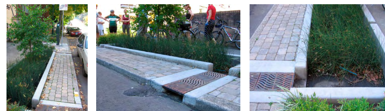
A curb cut channels street runoff into structured planters, where it is allowed to percolate into the soil
