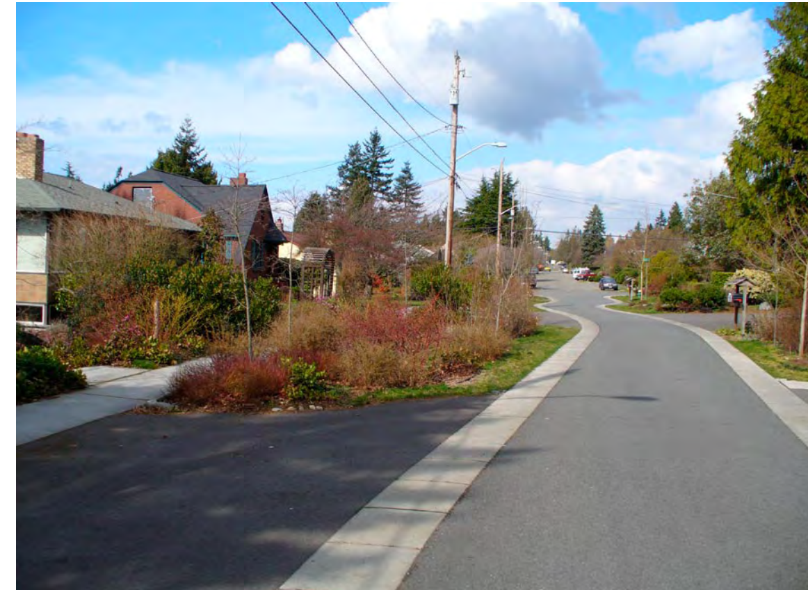
Curbless green streets are often found in residential areas. In this example, the green street treatment acts as a buffer between the sidewalk and roadway, and provides an amenity for adjacent homes
