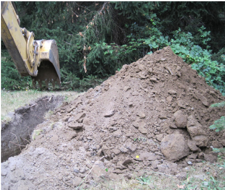
Photograph 4: Test pit TP-2 excavated material
