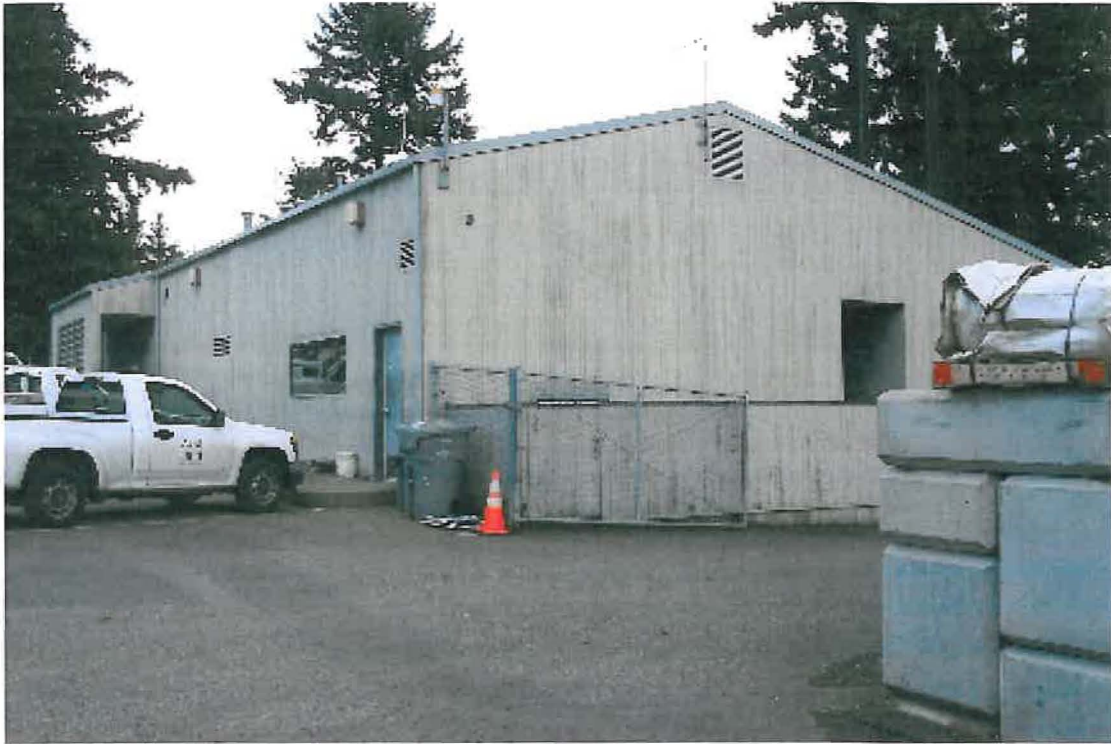
Administration Building – Looking Northeast
