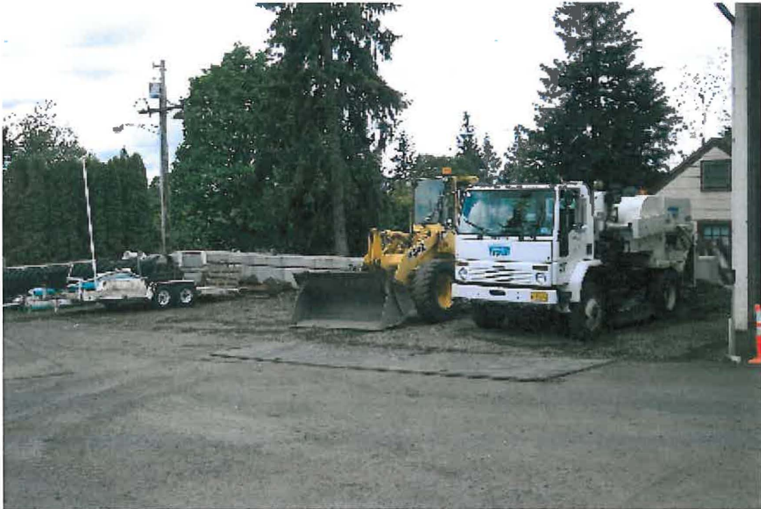
Covered Parking Building Site – Looking Southeast
