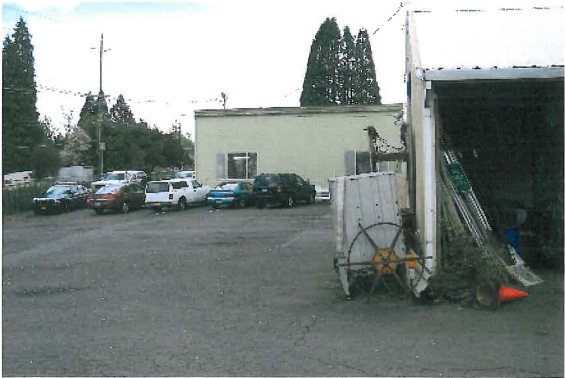
Vehicle Maintenance Shops – Looking North
