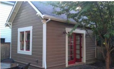
This accessory structure is an example of a compatible, not in period building. Its massing and height are similar to historic structures in the neighborhood. It has double hung wood windows and brackets in the gable ends, which are both common in the district.
