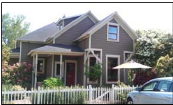
After, the artificial siding was removed and the historic wood siding and trim repaired and replaced, as needed.
