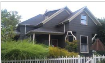
Before: Artificial siding was added over the historic wood siding and the trim altered and removed.
