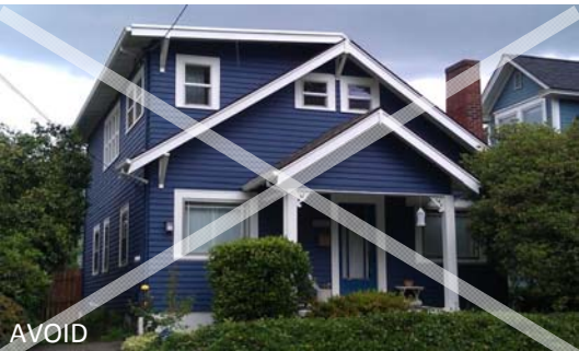
Incompatible addition that alters the roof pitch, is flush with the side elevation, and overwhelms the original residence.
