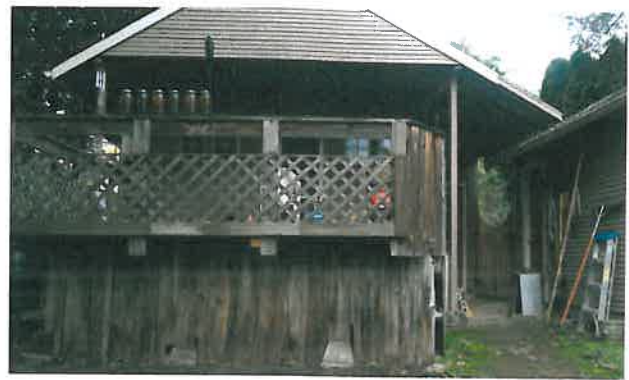
Existing rear addition and deck
