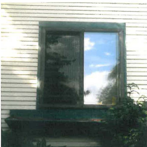
Aluminum window on the side façade
