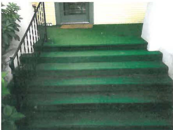
Front porch, carpeted stairs
