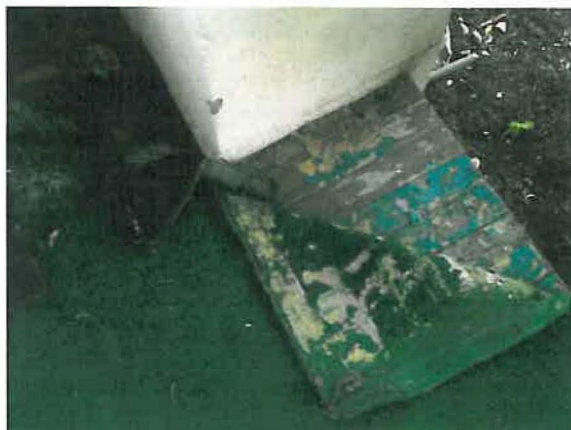
Front porch, under carpeting
