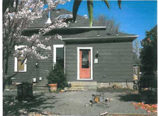
Rear elevation, restored shiplap siding visible on left
