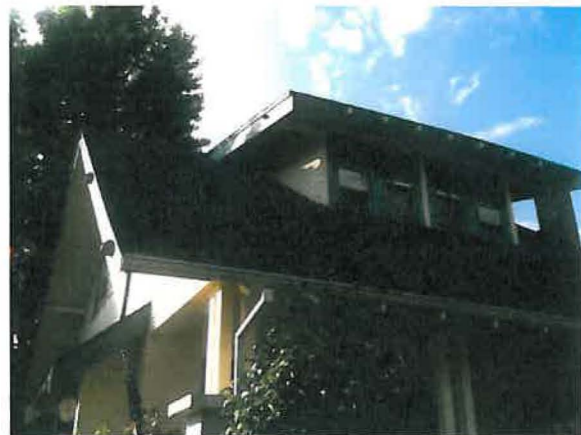
Front/Side elevations, brackets/corbels
