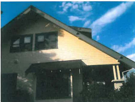
Side elevation, brackets/corbels
