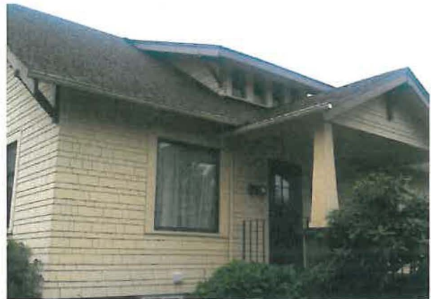
Front elevation, gutters
