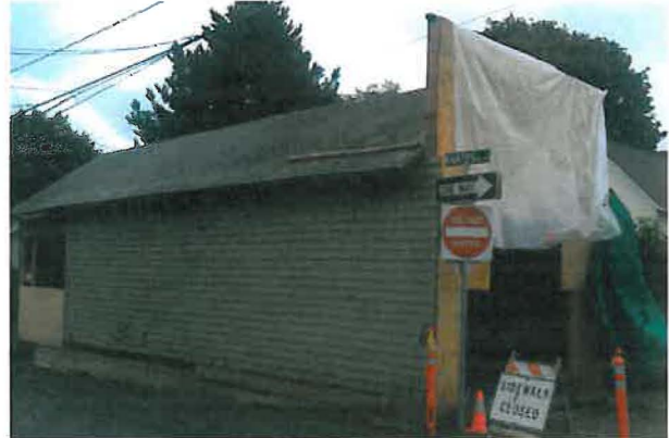
Accessory structure, work in progress
