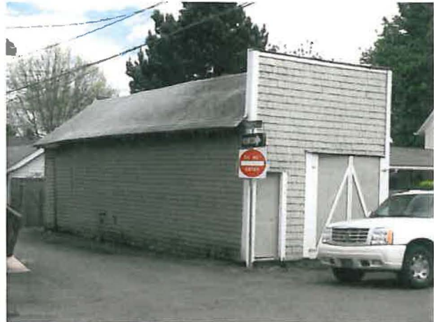
Accessory structure in rear yard, view from 13 th Street and Knapps Alley
