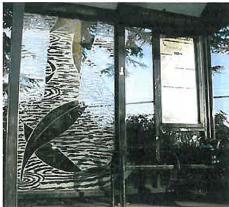
Sandblasting vandalized glass beautifies bus stops and deters further vandalism.
