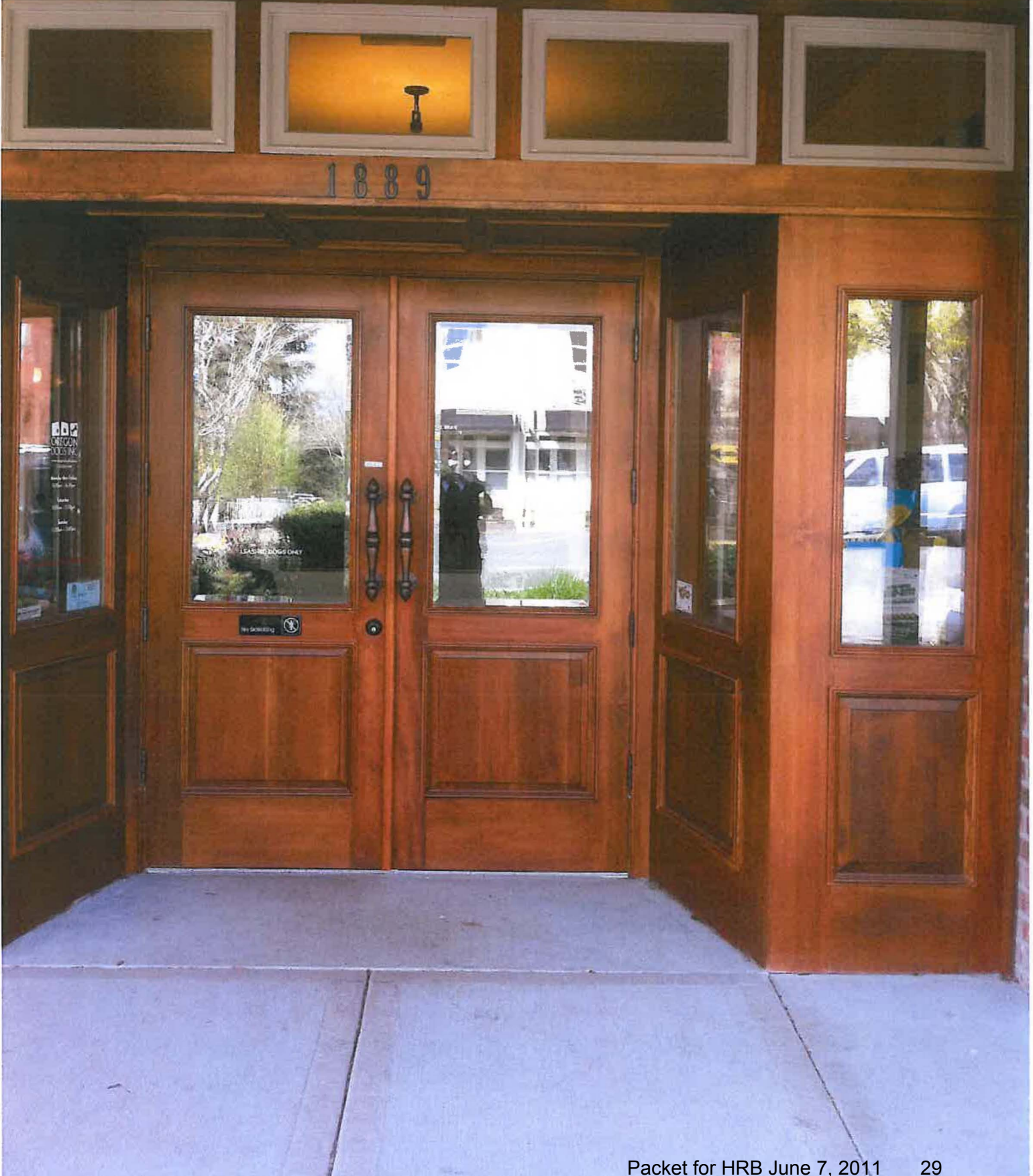
Photo #5 – 1823 proposed doors and stained window/door trim
